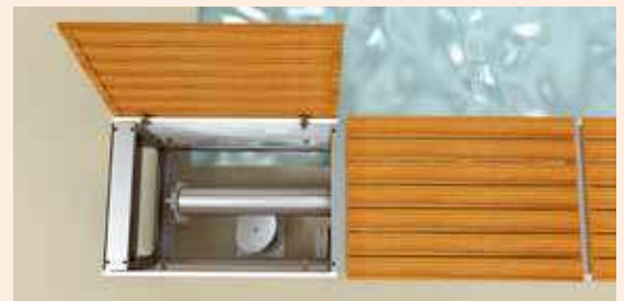
Access to the skimmers and mechanical parts
